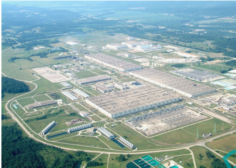
Aerial photo of the Portsmouth Gaseous Diffusion Plant showing the three large process buildings (center of photo) and other support facilities, facing southwest
